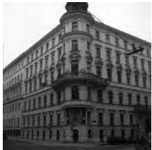
The OeAD on Campus Vienna The new OeAD House
